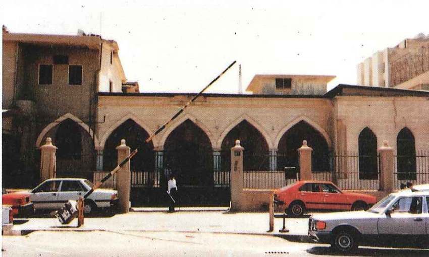
Fig.4 NORTH ELEVATION BEFORE RENOVATION
