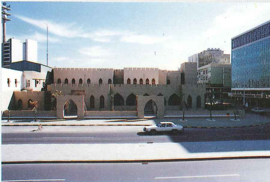
Fig.8 NORTH ELEVATION AFTER RENOVATION
